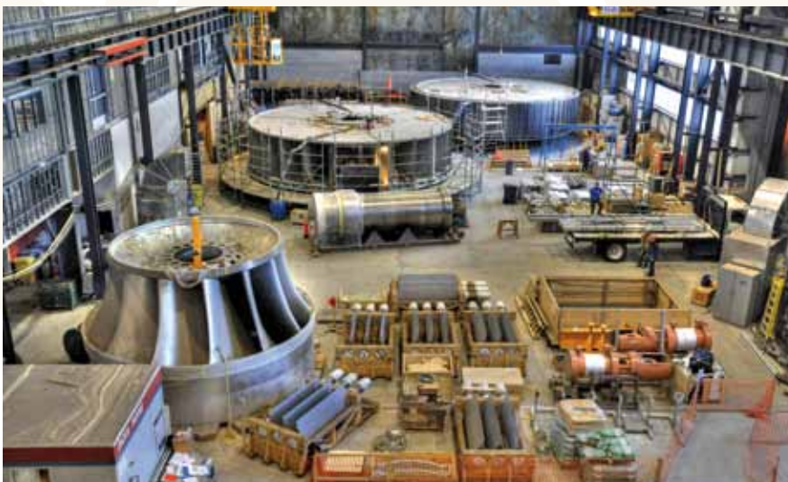
▲ Interior of Eastmain-1-A powerhouse during construction.
