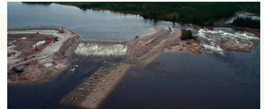
▲ Weir at KP 290 of the Rupert and channel allowing the free movement of fish.
