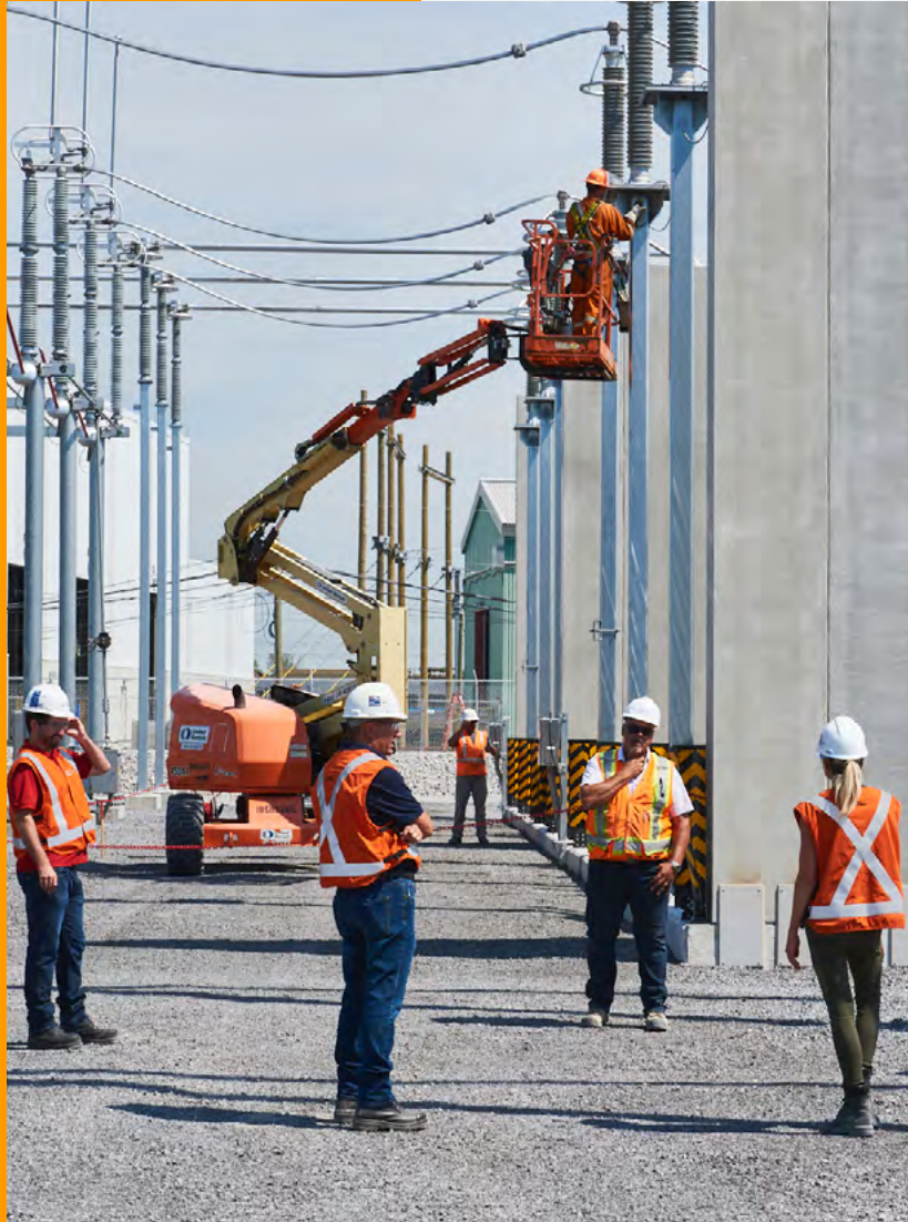
Preventive measures related to COVID-19 at the 315/25-kV Patriotes substation in Saint-Eustache. Pierre-Alexandre Bernier-Dionne, Manager - Construction, Pascal Monette, Manager - Projects, Yves Horth, Advisor - Safety, and Annie Giguère, Manager - Construction of Transmission Projects
