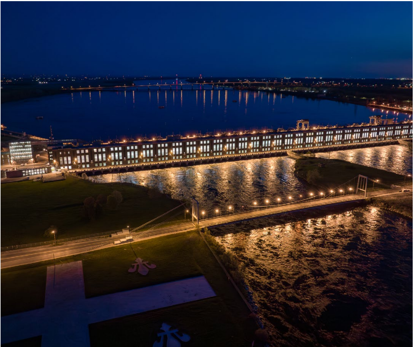
Beauharnois generating station.
